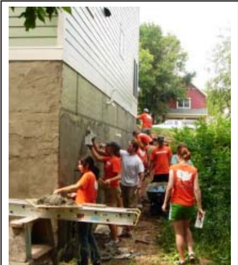
Bike & Build crews stucco a foundation on the new Lincoln Park homes.
