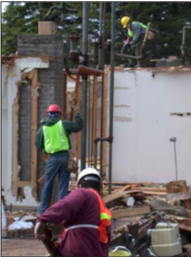
Common Ground Deconstruction crew members taking down a garage in Duluth.
